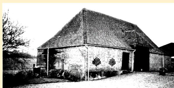
The eighteenth-century brick barn before the 2008 rebuild
